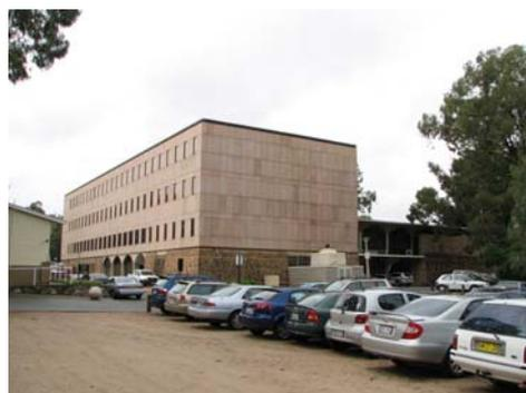
**Figure 4.3:** The northern block sits on the same stone plinth as the south block. Both north and southern faces are lined with aluminium or bronze framed windows. Views are of the front (above) and rear of the north block.
