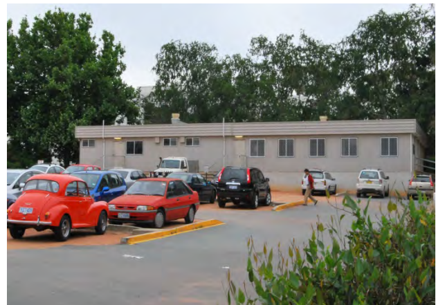
Figure 6: Demountable buildings connected to the north of the School of Art. (Source: ANU Heritage Office 2011)
