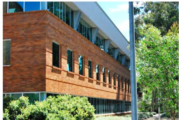
Figure 6: View of the CSIT Building with the combination brick metal construction type. (Source: ANU Heritage Office 2012)
