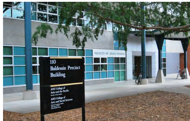
Figure 10: Main entrance to the Asian Studies Building. (Source: GML 2011)
