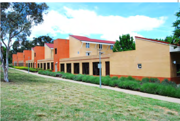
Figure 9: Eastern wall of (New) Graduate House, including gardens and walkway. (Source: ANU Heritage Office 2011)
