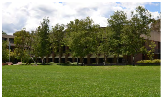
Figure 10: The western façade of Melville Hall, with its row of Populus alba . (Source: Heritage Office 2011)
