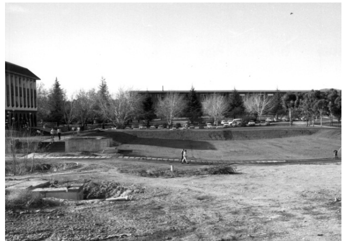
Figure 8: The site of the AD Hope Building from the south as photographed on May 7, 1965. (Source: ANU Archives)
