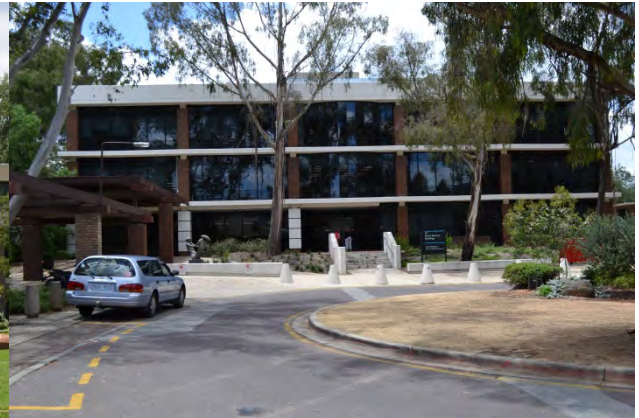
Figure 6: The entrance to the Beryl Rawson Building. The overarching walkway is visible to the left. (Source: Heritage Office 2011)
