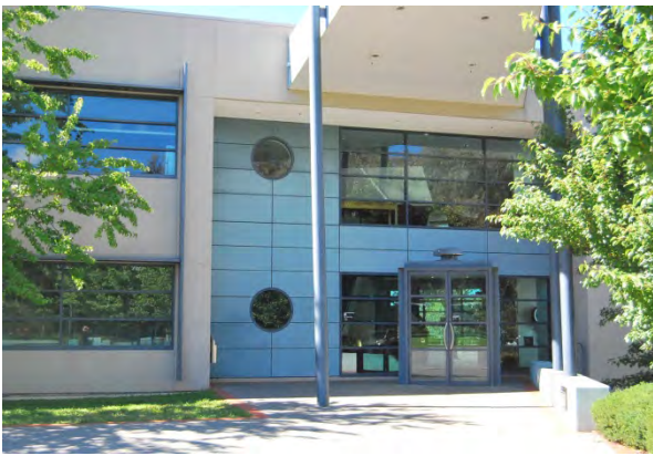
Figure 5: Front Entrance to the Sir Roland Wilson Building including airlock style doors. (Source: ANU Heritage Office 2011)
