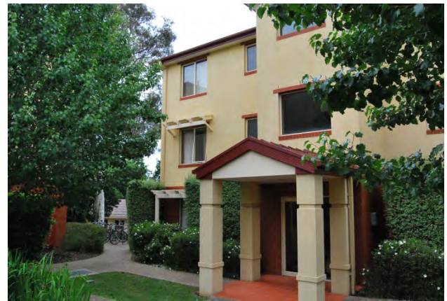
Figure 6: Front entrance to Block 5 including portico, wooden window features and examples of window styles. (Source: ANU Heritage Office.)
