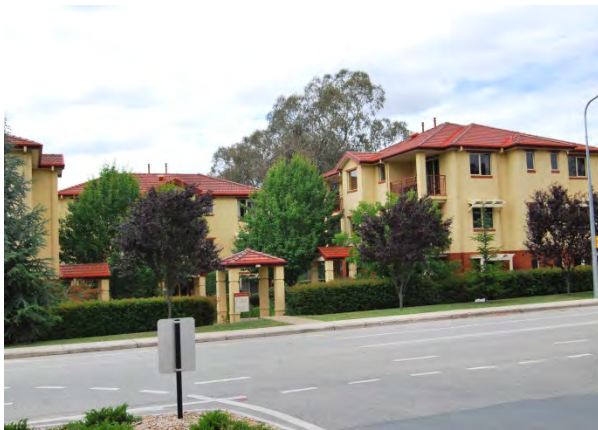
Figure 5: Front Entrance to Judith Wright Court including portico. (Source: ANU Heritage Office 2011)
