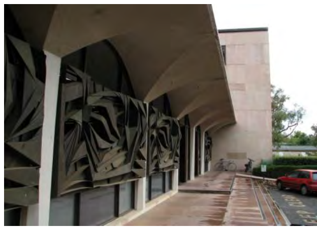
Figure 8: View of Dadswell Screens on the main entrance to the RG Menzies Building. (Source: ANU Heritage Office 2011)
