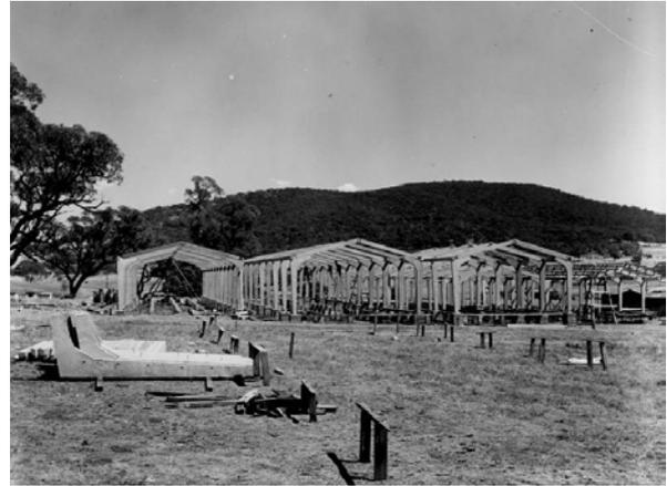
**Figure 6:** Construction of the temporary Medical School research facility, 4 March 1951. Note the concrete portal frames. (Source: ANU Archives)
