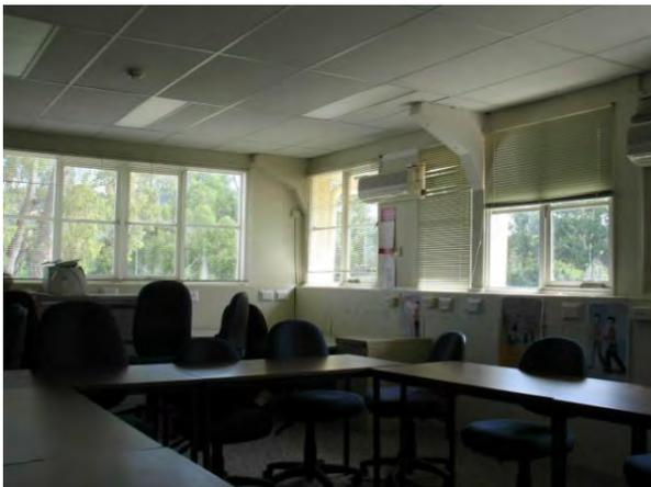
Figure 11: H Block, interior view showing exposed concrete portal frames. (Source: GML 2011)
