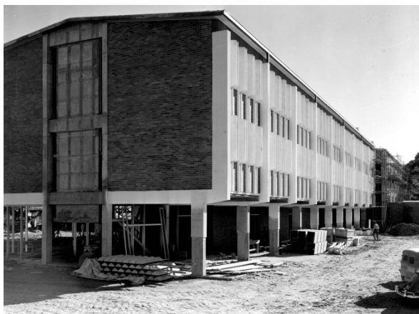
Figure 5: View of the Chemistry Building near completion April 1962. (Source: ANU Archives)
