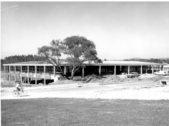
Figure 5: Construction of the Banks Wing (44) of BoZo, February 1964. (Source: ANU Archives)
