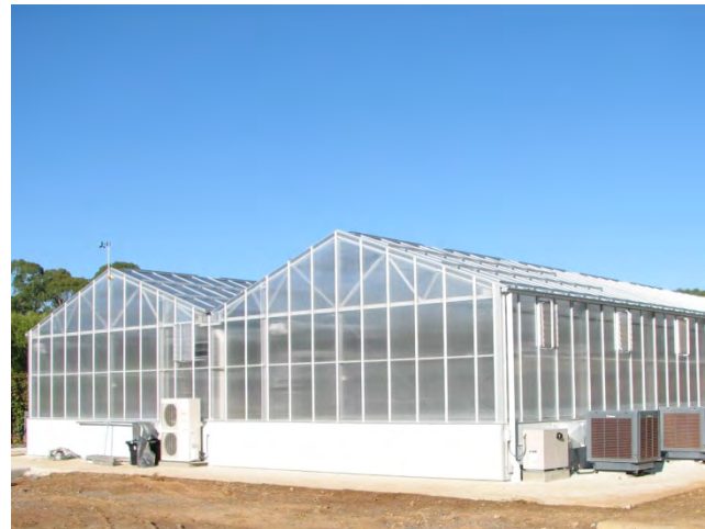
Figure 8: View of the New Glasshouses for the RSB. (Source: ANU Heritage Office 2010)
