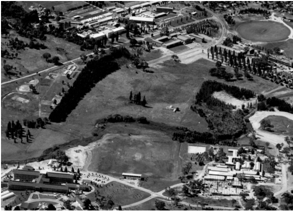
Figure 5: An aerial view of the RSB site circa 1951 including the Magnetic Hut, since demolished. (Source: ANU Archives)
