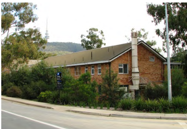
Figure 5: View of the ABE from the corner of Garran Road and Ward Road, pre demolition. (Source: ANU Heritage Office 2010)
