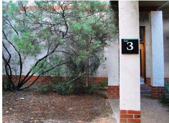
**Figure 10:** View of Entrance to Jaeger 3 featuring decorative brickwork and render combination on the building's exterior. (Source: ANU Heritage Office 2012)
