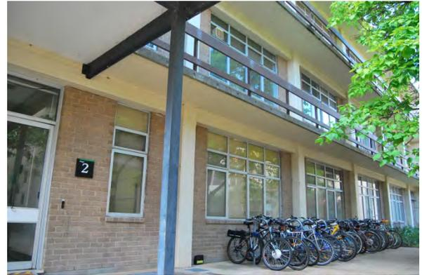
Figure 6: View of Jaeger 2 including concrete balconies and exposed brickwork. (Source: ANU Heritage Office 2012)
