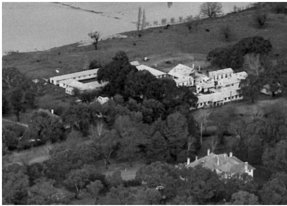
Figure 5: Construction of Block A, the Administrative Building, 1948. (Source: ANU Archives)
