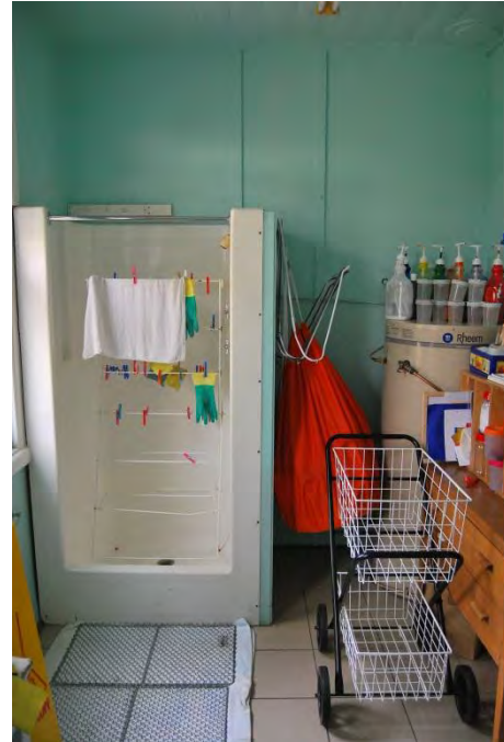
Figure 10: Original bathroom/laundry with original fittings. (Source: Heritage Office 2012)
