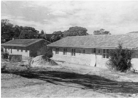
Figure 7: Brian Lewis Crescent houses under construction in 1952. (Source: ANU Archives)
