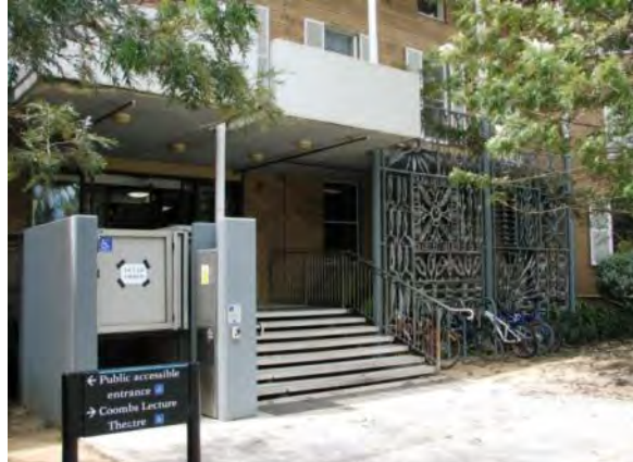
Figure 12: Southern view of the main entrance to HC Coombs Building. (Source: ANU Heritage Office 2011)
