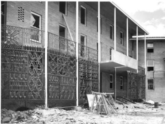
Figure 11: Main Entrance to the H C Coombs Building under construction with Skipper's Screens Installed. 1963. (Source: ANU Archives)
