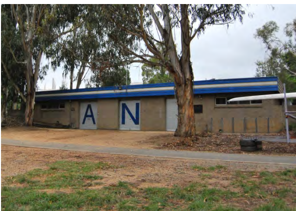
Figure 5: Western façade of the ANU Boathouse with roller doors and bicycle racks. (Source: ANU Heritage Office 2012)
