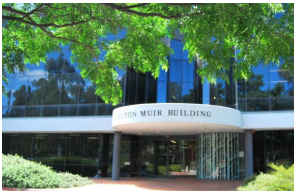
Figure 5: Front Entrance of the Fulton Muir Building including frosted feature window. (Source: ANU Heritage Office 2012)
