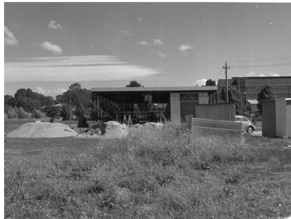
Figure 10: South Oval Sports Pavilion Under Construction 1965 (Source: ANU Archives)
